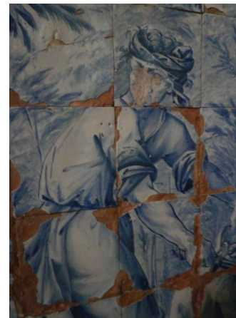
Figure 2. Effect of decay. Glaze lacunae at the edges of the tiles.
