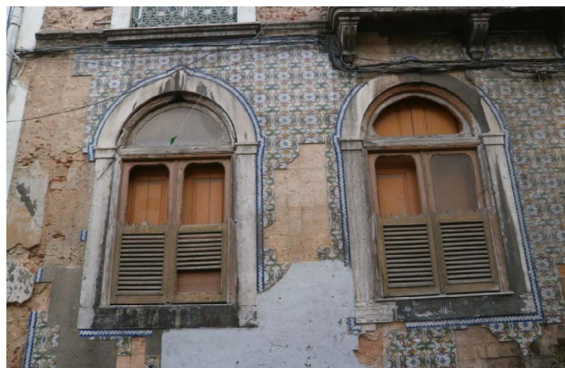
Figure 2. Lack of maintenance, loss of tiles and unappropriated interventions.
