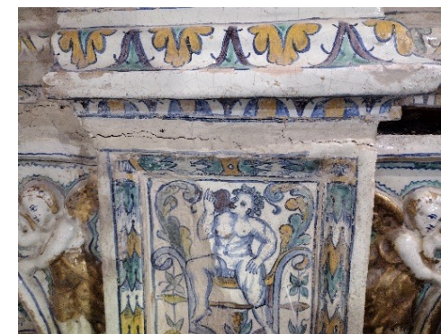
Figure 1. Grout damages detail.
